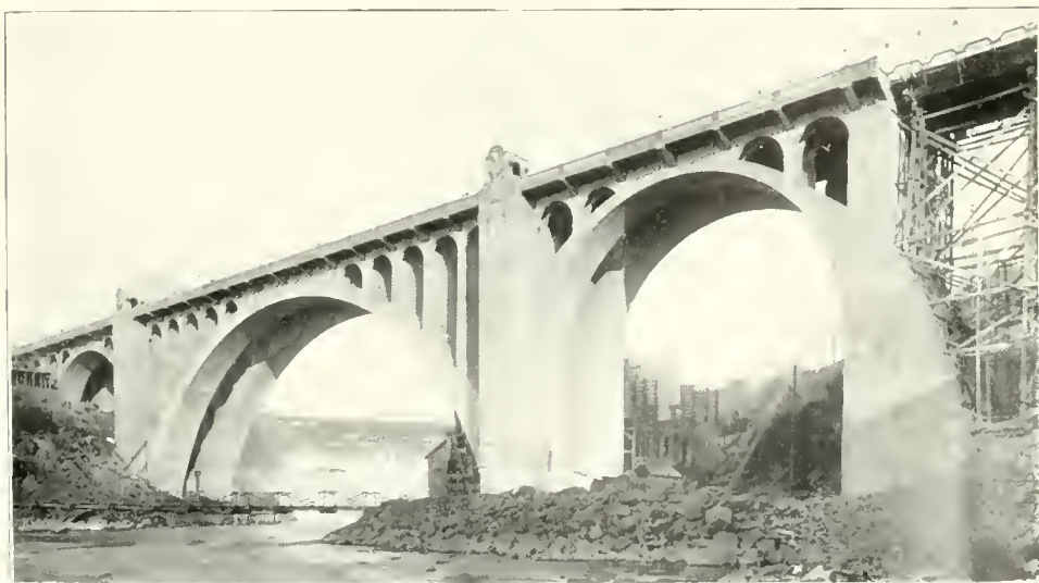
NEW MONROE STREET BRIDGE, COMPLETED IN 1911 AT A COST OF FIVE HUNDRED THOUSAND DOLLARS. LONGEST CONCRETE ARCH IN THE UNITED STATES
